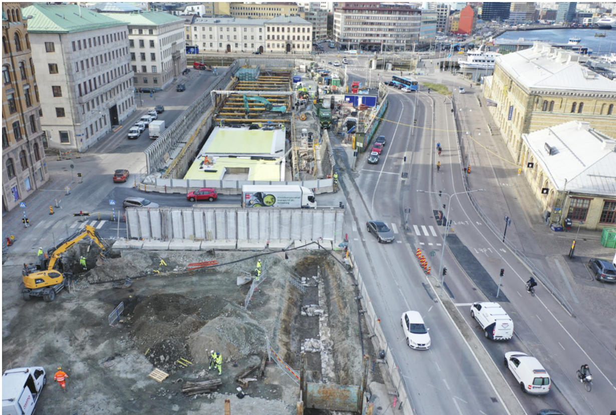
Fig. 10. Excavation work taking place in part of the Kvarnberget area. A section of a curtain wall with counter-foots can be seen near the centre of the picture. It is a good illustration of how the excavations were carried out in the middle of a busy town. Photo: Arkeologerna. Photo: Arkeologerna.
