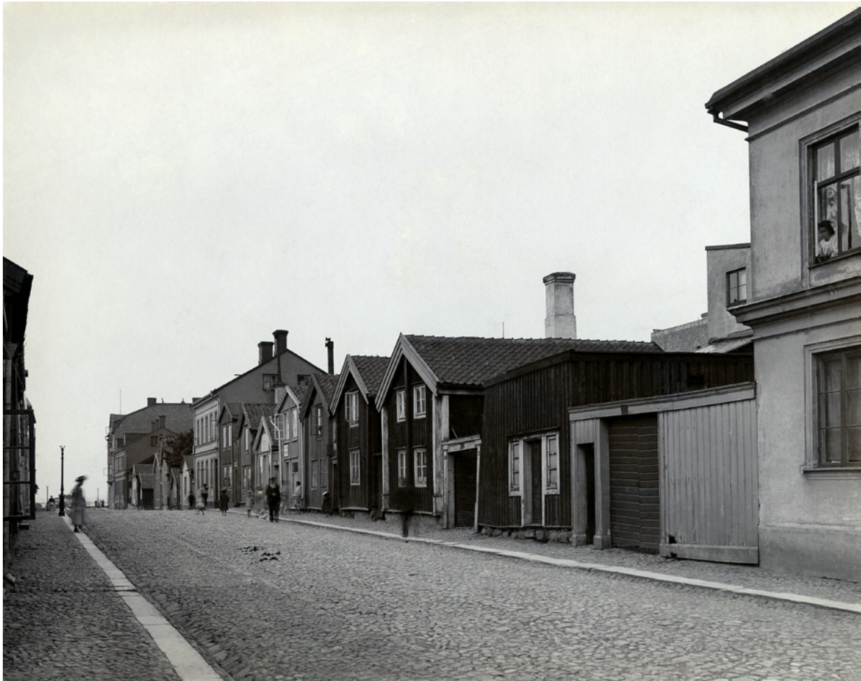
Fig. 6. A section of Norra Långgatan, Kalmar. Houses with the gable end facing the street, and a high wooden fence with a door leading into the narrow yard. Every house and plot has its specific life course and biography – a challenge and an opportunity. Photo Archive of Kalmar läns museum.
