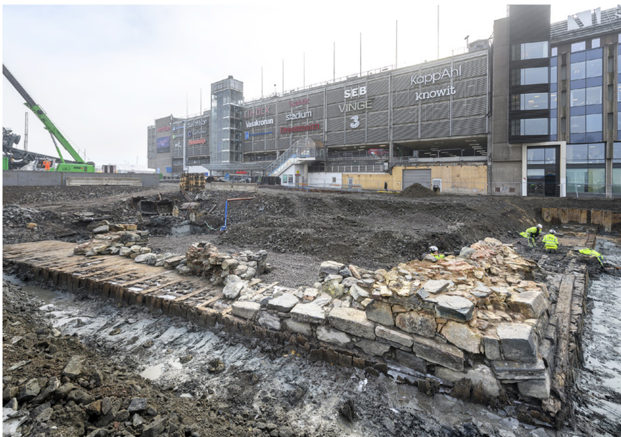
Fig. 9. The western side of the bastion Gustavus Primus, with a stonewall and wooden foundation. Photo: Markus Andersson for Arkeologerna.
